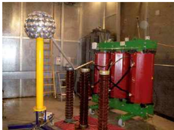
Partial discharges test at CESI (MI)
